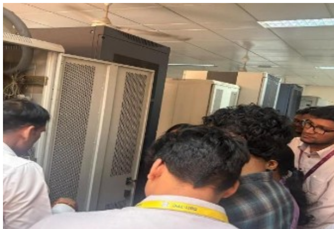
Photo 4: Visit to the telecommunication and networking equipment area.
